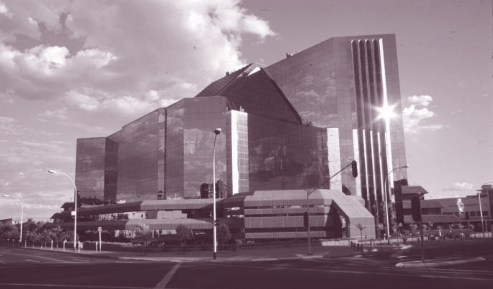
MANGAUNG LOCAL MUNICIPALITY (BLOEMFONTEIN): NEW CIVIC CENTRE EXTERIOR. ©KEITH YOUNG/IAFRIKA PHOTOS
